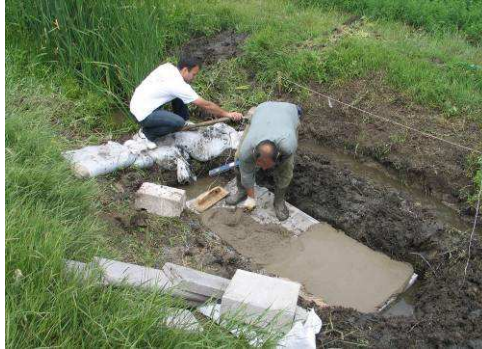
Incorporation of access tube
