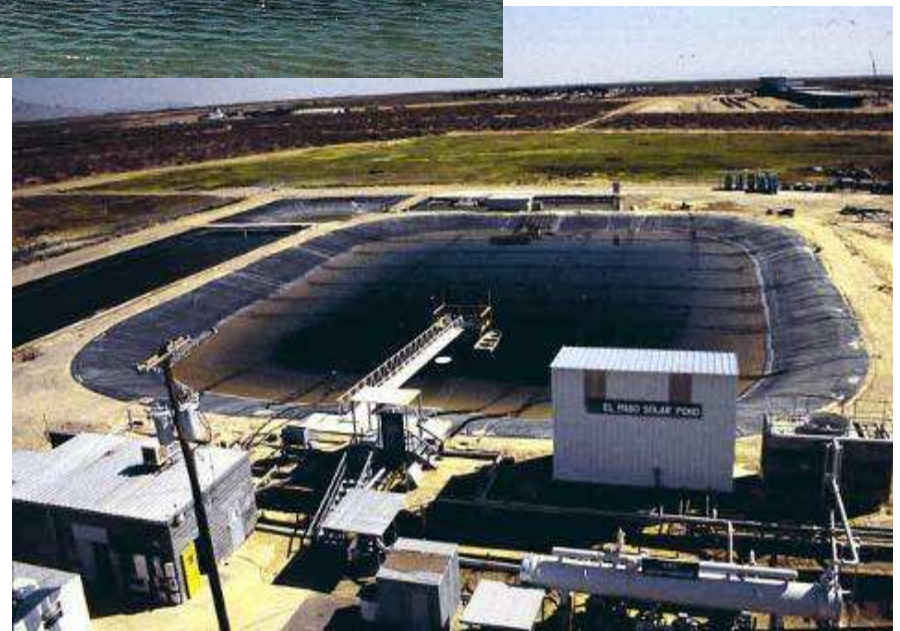
Solar Ponds at El Paso (Texas) → one of 210,000 m 2 and another of 1,900,000 m 2
