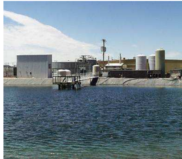
Solar Ponds at El Paso (Texas) → one of 210,000 m 2 and another of 1,900,000 m 2
