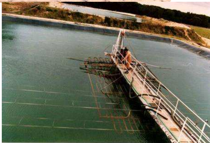
Solar Ponds near Lisbon (Portugal) → 1024 m 2 with heat exchanger at the bottom
