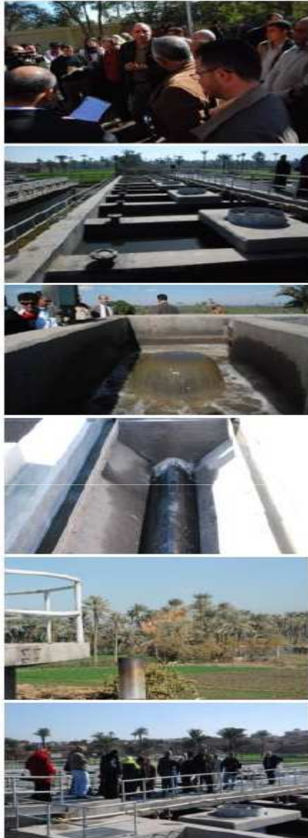
The First UASB WWTP Sanhour, Fayoum Governorate
