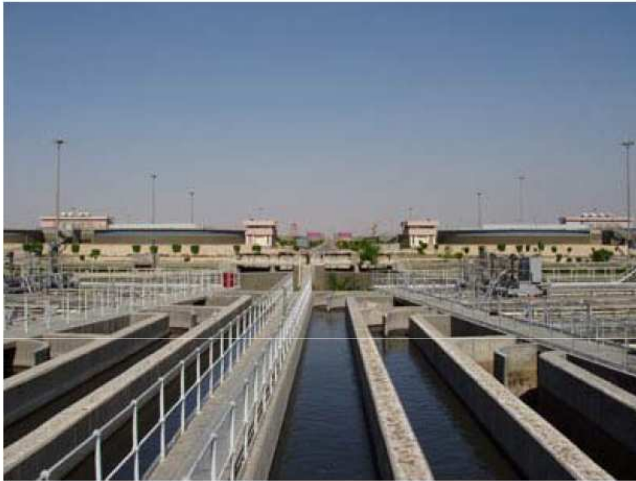
The Gabal El Asfar WWTP. The picture is taken from one end of the area and the two purple biogas towers in the middle of the picture is about 2 kilometres away! The plant is getting even bigger by further construction work and 2007 it will serve 12 million people.
