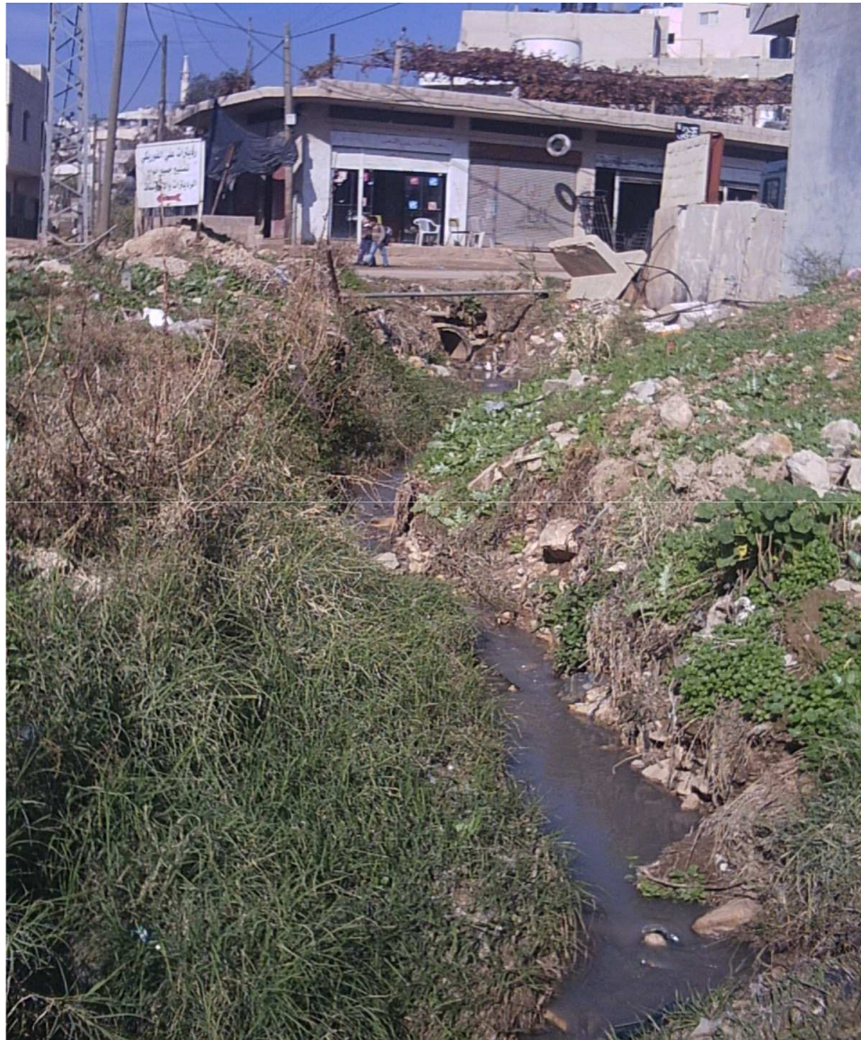
Gray wastewater stream discharged through open channels from Al-Fara Refuge Camp.
